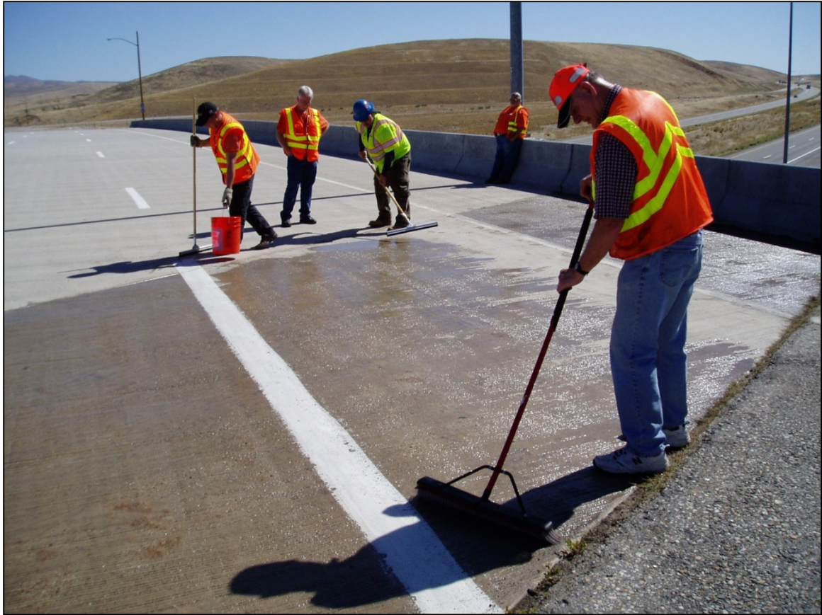
Figure 4.5 East Eisenmann Bridge Site
